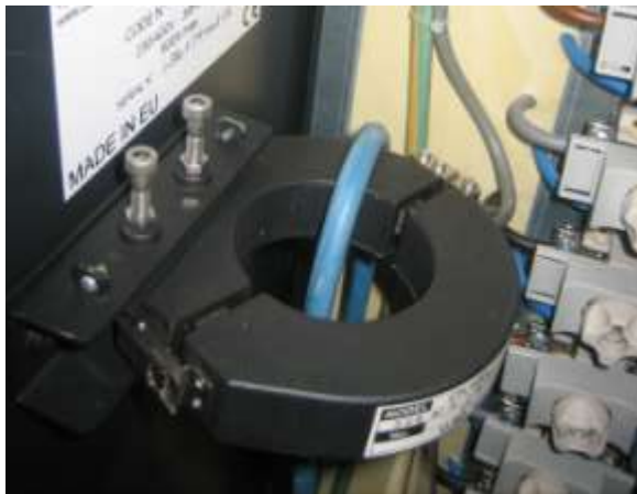
Detail of TI with mounting Kit
